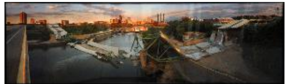
The disastrously pancaked I-35W bridge is the haunting centerpiece of a panoramic vista of Minneapolis' skyline in Chuck Arnold's photo "Collapse."
